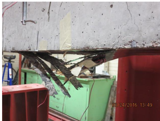
Failure of Beam
